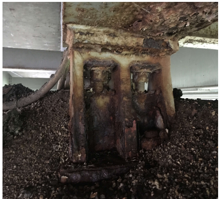
PHOTO 2 Description Fixed bearing condition at bent #2. Typical of bearings # 4-6.
