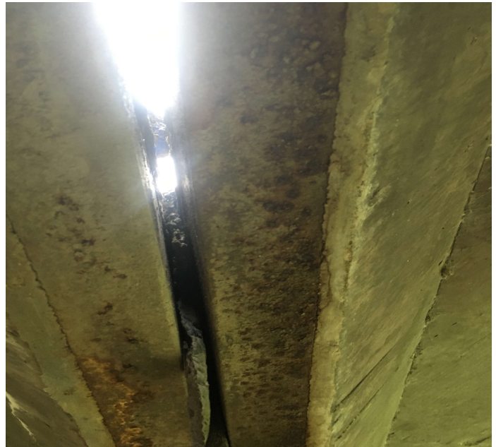
PHOTO 2 Description Areas of Missing joint seal over bent #5 allowing free flow of water.
