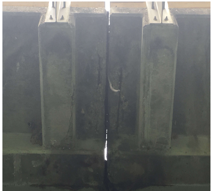
PHOTO 2 Description Shallow rebar exposed on the underside on the right concrete bridge rail in spans #5,6.
