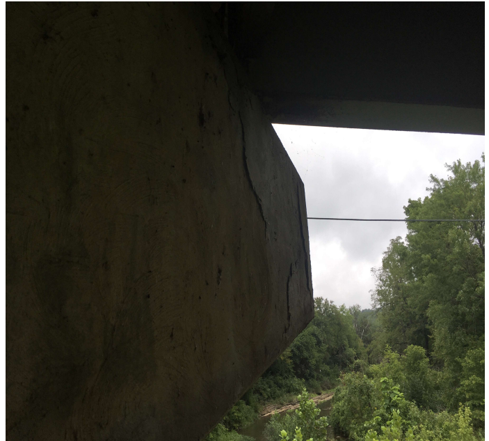
PHOTO 2 Description Large delaminations on the span #5 side of the bent #4 cap. Typical of the left and right sides.
