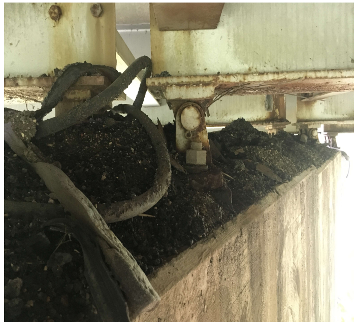
PHOTO 2 Description Heavy build up on the bent #5 cap.
