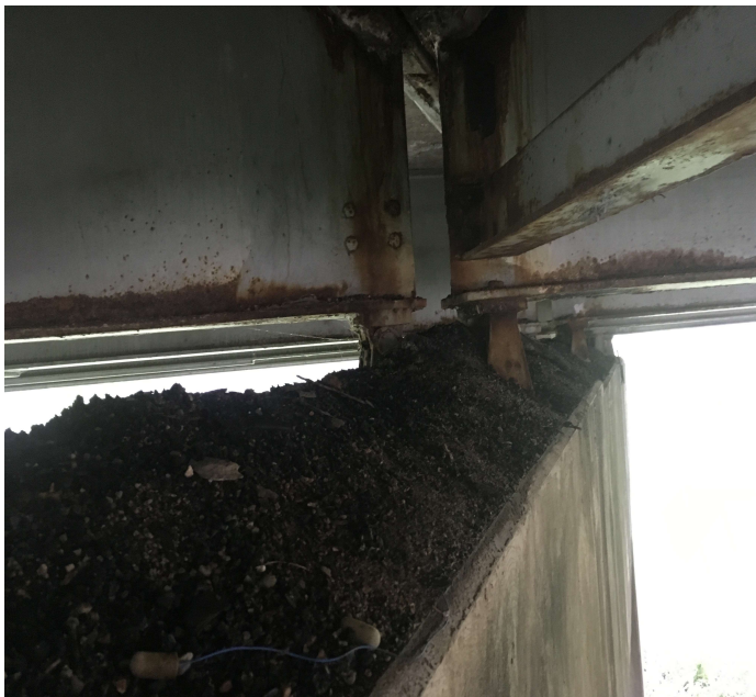
PHOTO 1 Description Heavy Debris build up on the bent #2 cap.
