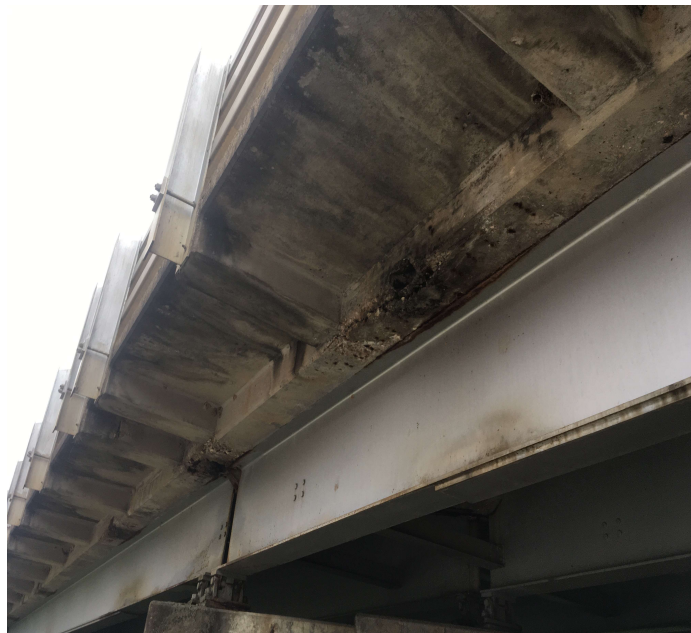
PHOTO 1 Description Drain area condition. Showing spalling and delamination some with rebar exposed. Typical of many locations.
